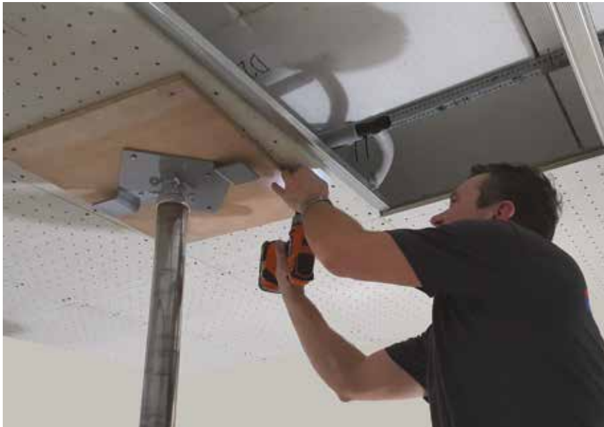
Montage von Deckenpaneelen Heating - cooling panels assembly
